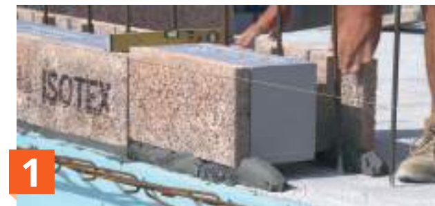
Laying of the first row with spirit level for levelling
