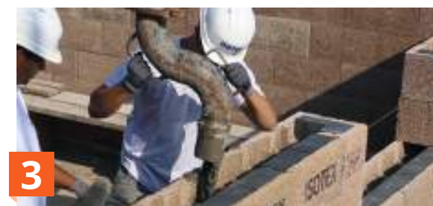
Filling of the blocks with concrete (every 6 rows)
