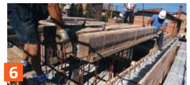
Laying of the floor slabs, calculated and made to measure.
